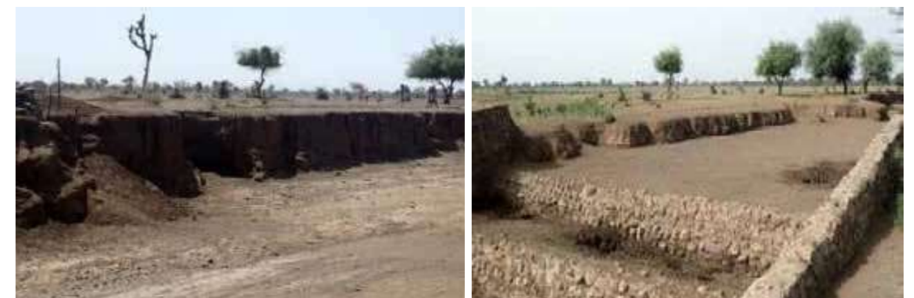
Figure 59: A water spreading weir successfully stopped erosion and trapped lost soil two years after construction (Photo DVRPU)
