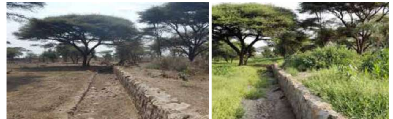
Figure 62: A water spreading weir shortly after construction (Photo DVRPU) Figure 63: The same weir one year later with grasses able to slow water velocity (Photo DVRPU)
