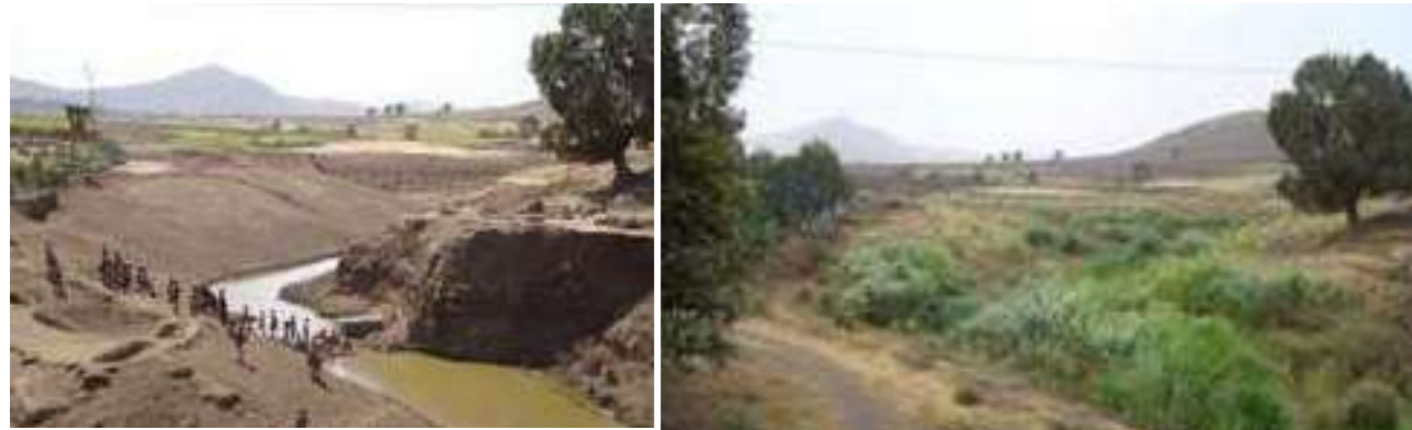
Figure 64: Zone 5 stabilising riverbanks with grasses, shrubs and fruit trees (Photo DVRPU)
