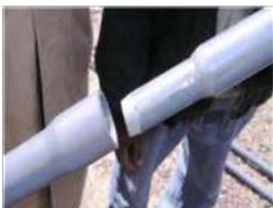
**Figure 3 – Creating a socket.** Heat up the end of the rising main. Insert the tool. Cool the end of the rising main with water (turn the tool around to prevent it from getting stuck). Remove the tool from the rising pipe. The socket is created.
