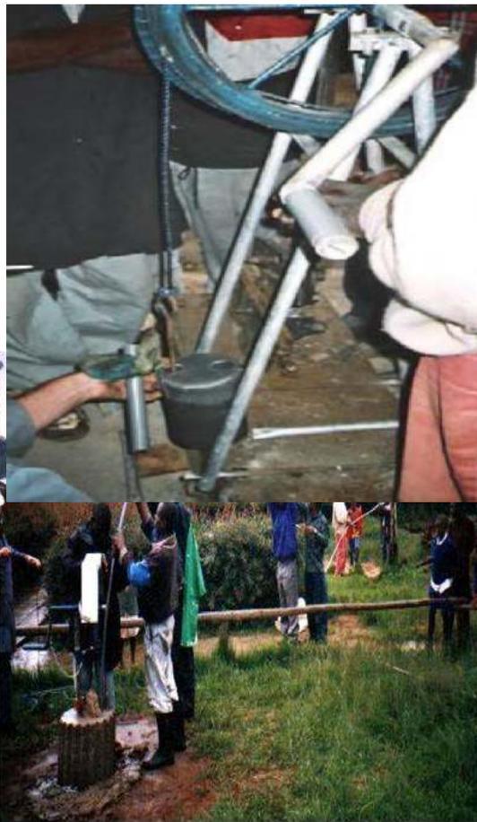
Mark the top end of the riser main on the side on which the catcher pipe of the guide box is to be situated. This is needed to ensure that the guide box (at the bottom) and the pump (on top) are properly aligned after installation. If this is not done carefully the rope and pistons might become entangled around the riser main and get stuck.
