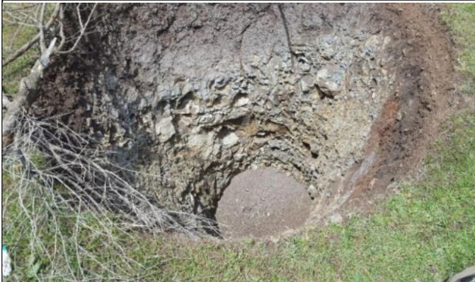
Figure 7. Percolation pit in gravelly soil - cascaded in a waterway
