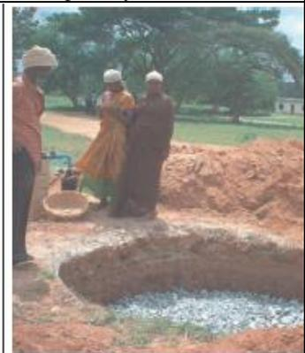
Figure 9. Excavation (left), backfilling with small stones and gravel (middle), and placement of coarse sand on top of the gravel
