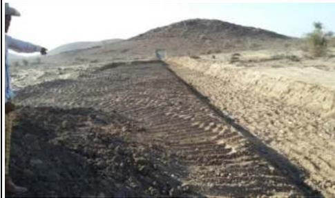
Cutoff wall construction and compaction
