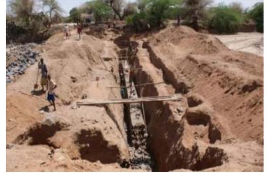
Fig 4. Subsurface dam under construction - Dire Dawa area, Ethiopia
