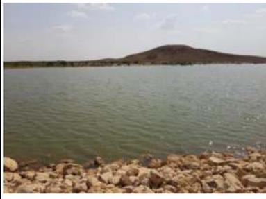
Scene of completed earthen dam, see the stone rip-rap on the upper side of the embankment
