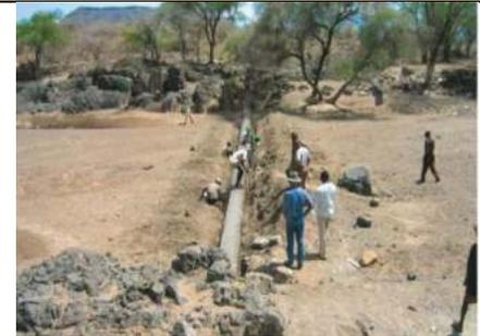
Fig 5. Subsurface dam under construction
