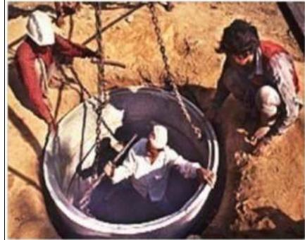
To make the construction of a hand-dug well viable, water must be available in sufficient quantities at shallow depths (6 to 25m) that will allow safe excavation and economically feasible exploitation of the water resources in the well. This will depend, of course, on local conditions, for instance it must have stable soil and a depth to the water table that does not allow pollution.
