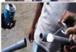
**Figure 4 – Making the connection.** Roughen up the inside of the female and the outside of the male part with sandpaper. Glue the pipes together. When glue the pipes together, only glue the male part. NOT the inside of the female part. If you do so, the male part will push the glue inside the female part forward, creating a rim on the inside, which could block the pistons.
