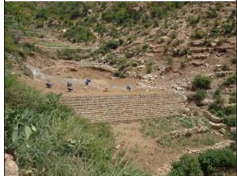
Fig.2 Sediment Storage dam Construction in diredawa - Beke-halo
